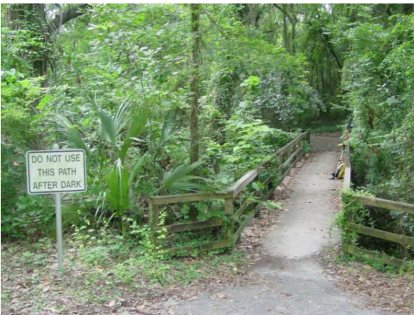
Bridge over Ravine's Creek
